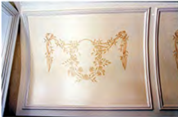
Monochromatic motif on barrel vault ceiling with painted plaster faux finish on walls
